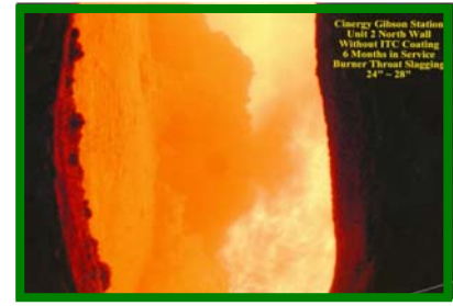
These are the burner throat and water wall before and after coating with technical ceramic materials.
