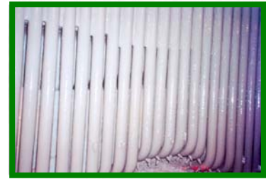
These are the burner throat and water wall before and after coating with technical ceramic materials.
