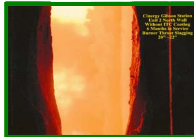
These are the burner throat and water wall before and after coating with technical ceramic materials.
