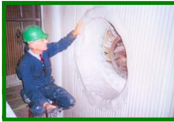
These are the burner throat and water wall before and after coating with technical ceramic materials.
